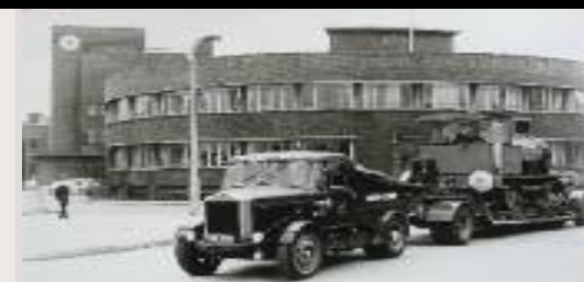
8 SHUNTERS AT SHEET WORKS Memories by Keith Atherton
